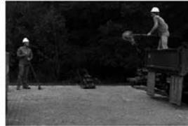
Figure 10. Spreading and sweeping joint sand.
