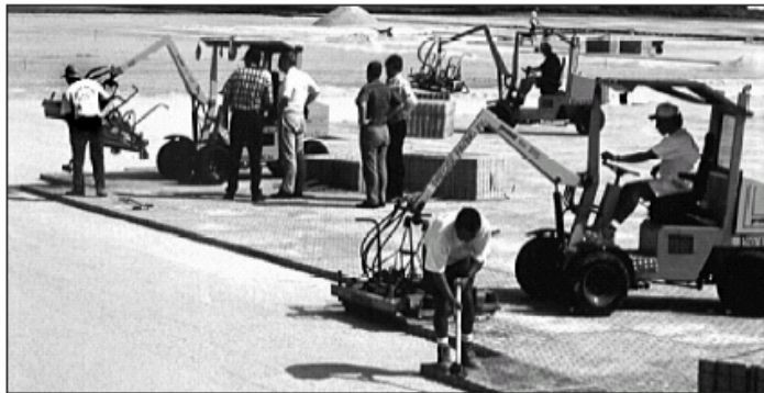
Mechanical installation equipment places concrete pavers rapidly.
