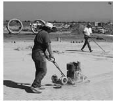
Figure 11. Vibrating sand into the joints.
