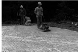
Figure 9. Compacting the pavers and bedding sand.
