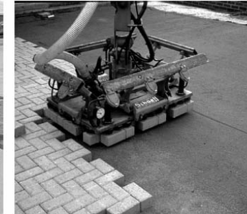
Figure 6. The vacuum head over the paver layer.
