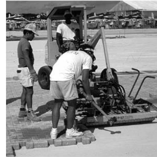
Figure 5. Motorized equipment with a hydraulic clamp.
