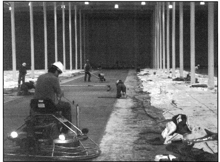
Floating, highway straight-edging and troweling of superflat slab Curve Lite Glass
