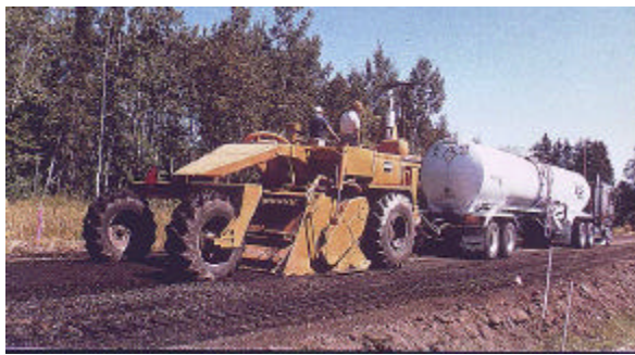
Figure 3-8.5. Soil stabilization mixing equipment for adding stabilizer.
