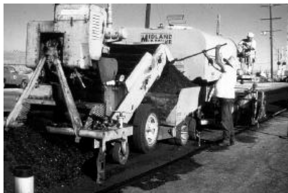
Figure 3-8.7. Traveling mixer using windrow elevator for recycled asphalt pavement pickup.
