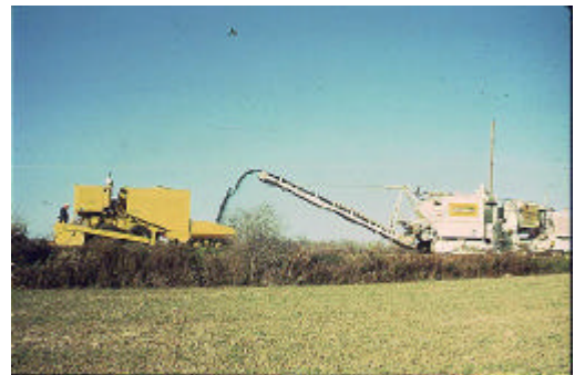
Figure 3-8.6. Traveling mixer adding stabilizer asphalt pavement form cold-milling machine.
