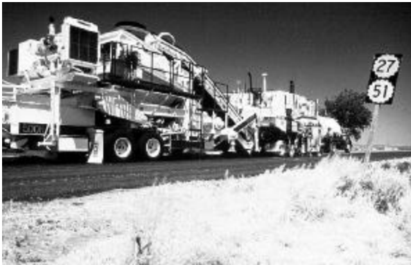
Figure 3-8.13. Portable crusher attached to cold-milling machine.
