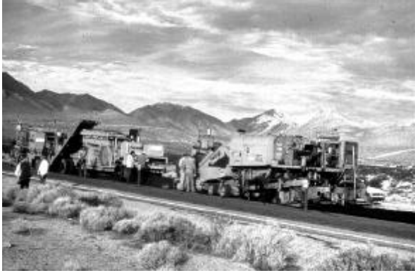
Figure 3-8.11. Single-pass equipment train.
