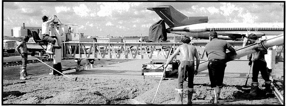
The C-450 is ideal for finishing airport aprons or any flat slab project.
