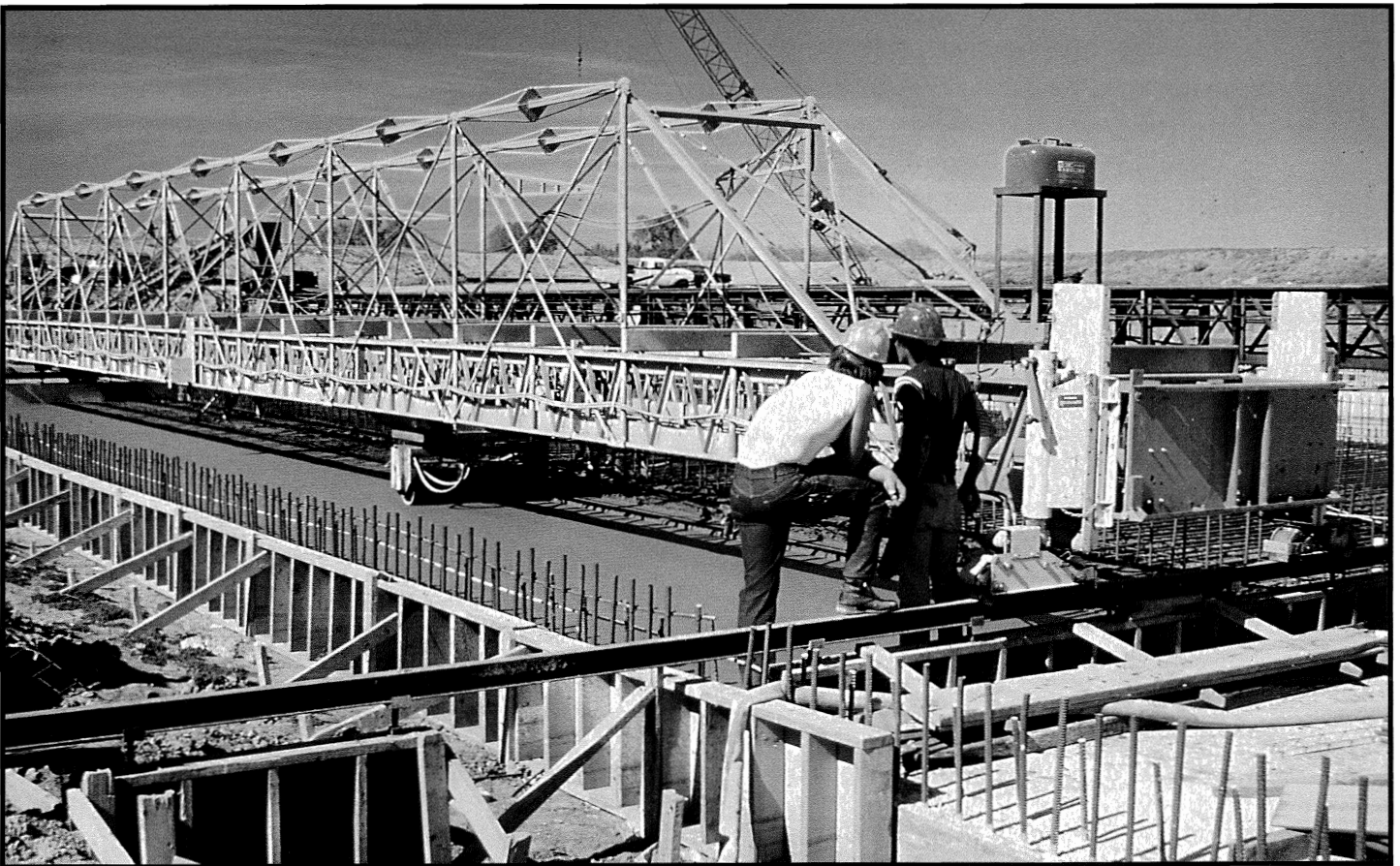
Self-Widening...The C-450's wide range of standard equipment includes self-widening jacks for automatic negotiation of tapered decks and slabs. Overhead Truss Assembly... By adding the overhead truss, you have the advantage of taking the basic 450 frame to wider widths and by removing the system, the basic 450 frame can be used for narrower width applications. This gives the GOMACO 450 model the versatility to adapt to several projects. GOMACO engineers recommend the truss system at widths exceeding 76 ft. (23.16 m).
