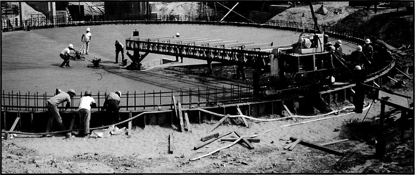
Pivot Point Operation...Waste treatment facilities which require a 360 degree concrete finish can easily be accomplished with the C-450 pivot point operation.
