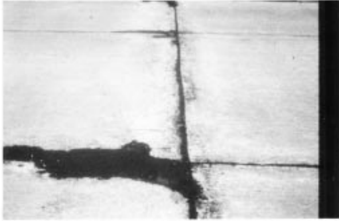
FIG. X2.45 Medium-Severity Scaling
