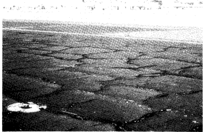
FIG. X1.19 High-Severity Block Cracking
