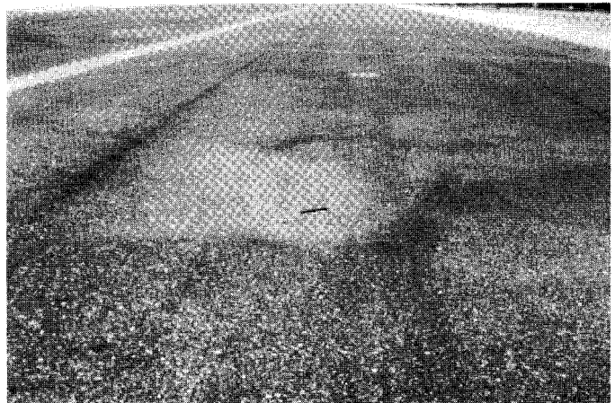
FIG. X1.26 Medium-Severity Depression
