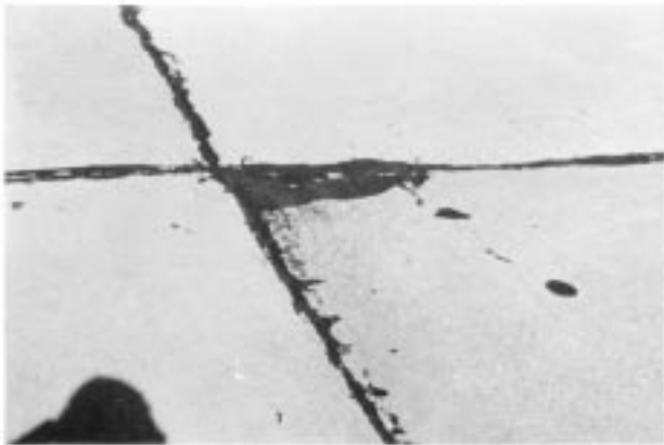
FIG. X2.19 Low-Severity "D" Cracking Approaching Medium Severity
