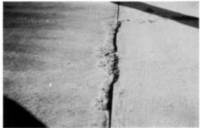
FIG. X2.68 High-Severity Joint Spall
