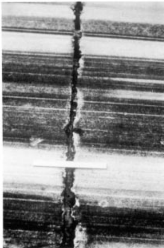
FIG. X2.62 Low-Severity Joint Spalling (if the Frayed Area was Less Than 2 ft (0.6 m) Long it Would not be Counted)
