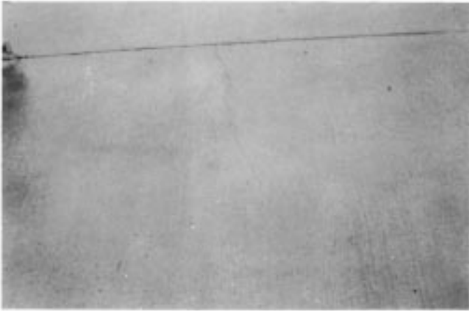
FIG. X2.61 Shrinkage Cracks
