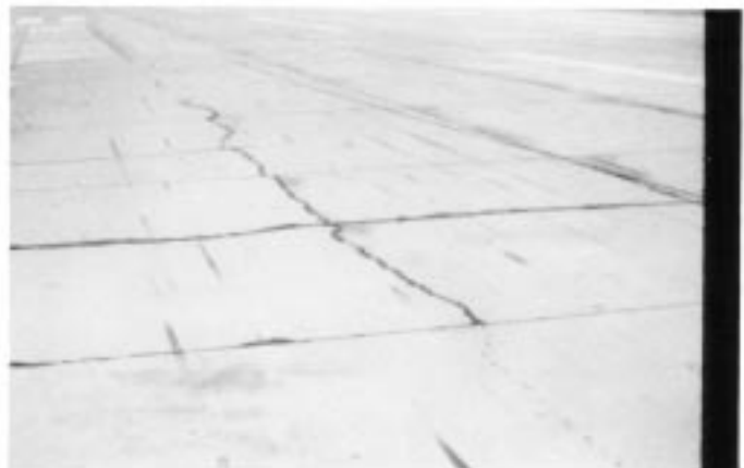
FIG. X2.54 Low-Severity Intersecting Cracks
