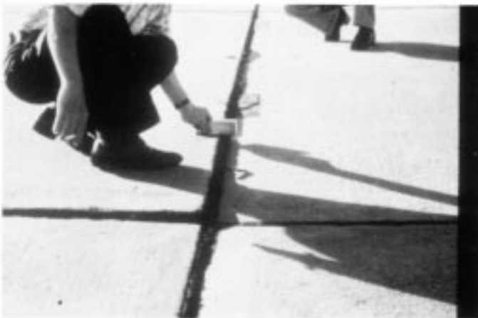
FIG. X2.53 High-Severity Settlement
