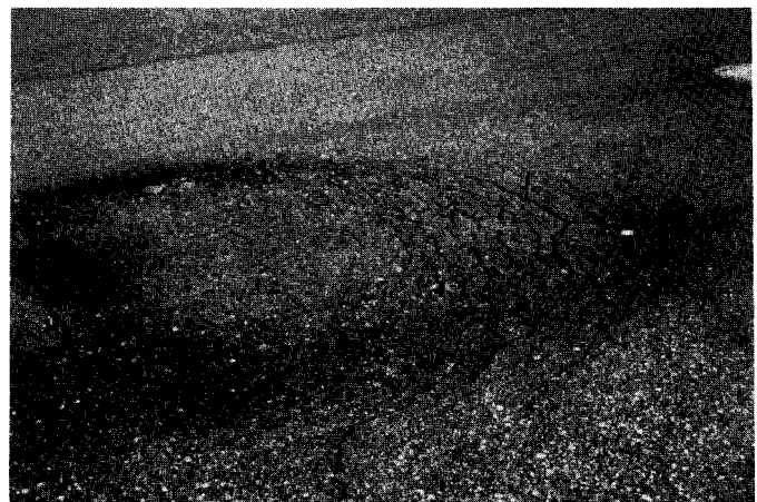
FIG. X1.73 Slippage Cracking
