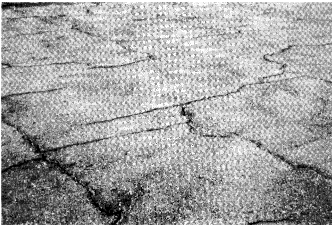
FIG. X1.17 Medium-Severity Block Cracking
