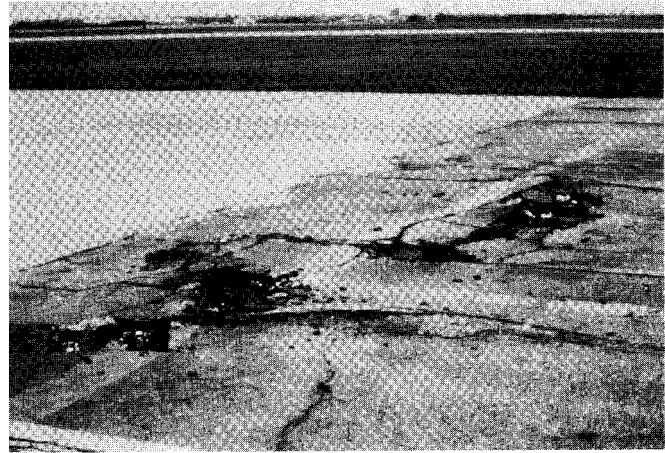
FIG. X1.72 High-Severity Shoving
