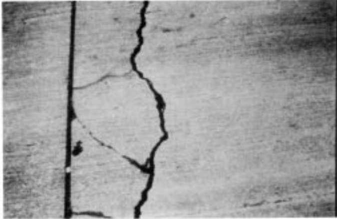
FIG. X2.65 Medium-Severity Joint Spall
