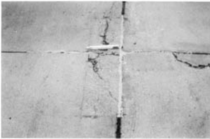
FIG. X2.32 High-Severity Small Patch
