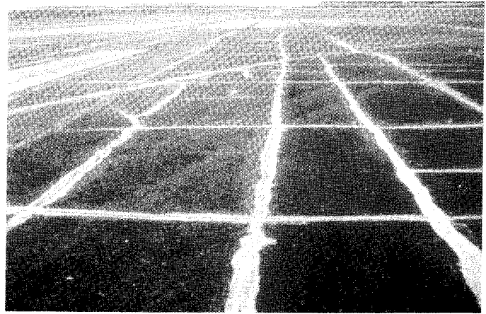
FIG. X1.13 Low-Severity Block Cracking, Filled Cracks
