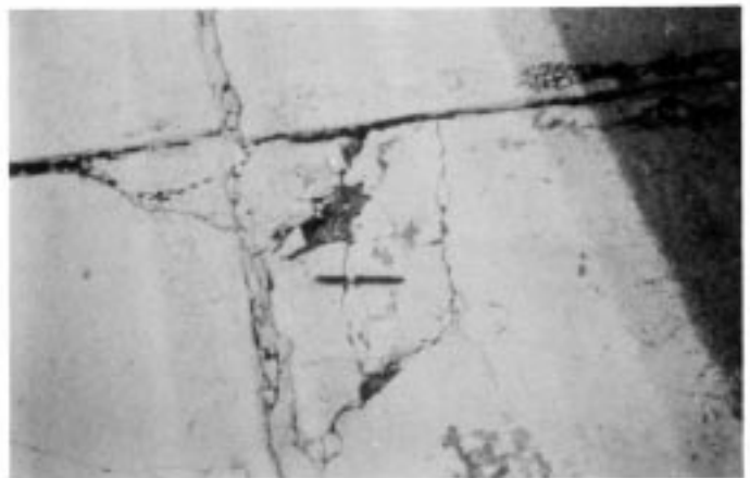
FIG. X2.74 High-Severity Corner Spall
