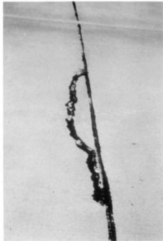
FIG. X2.63 Low-Severity Joint Spall
