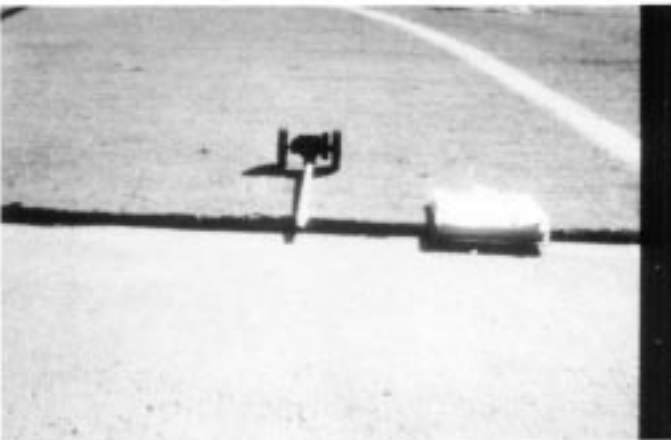
FIG. X2.52 High-Severity Settlement on Taxiway/Runway (¾ in. (18 mm))
