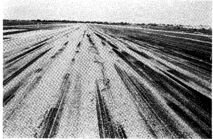
FIG. X1.38 Low-Severity Longitudinal Cracks, Approaching Medium
