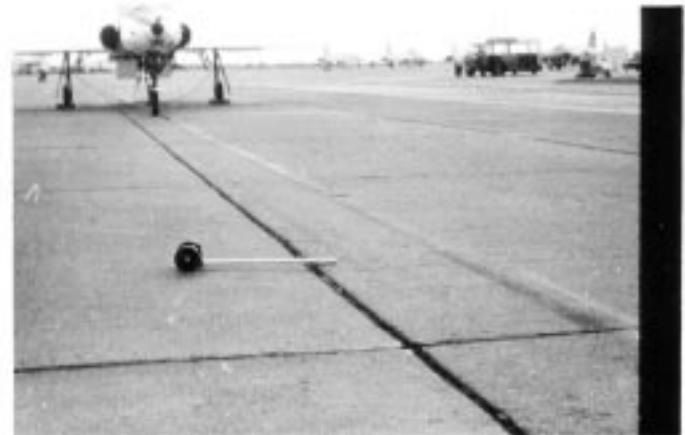
FIG. X2.50 Low-Severity Settlement on Apron
