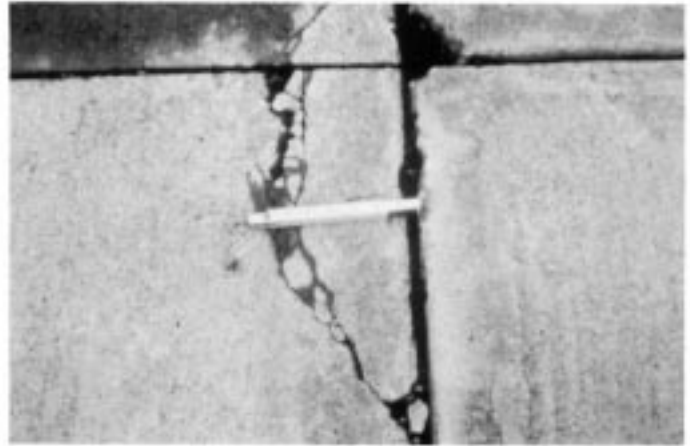
FIG. X2.72 Medium-Severity Corner Spall
