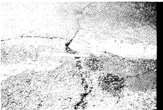
FIG. X1.42 High-Severity Longitudinal Crack
