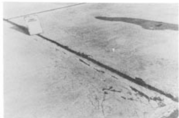
FIG. X2.21 Medium-Severity "D" Cracking Occurring in Limited Area of Slab
