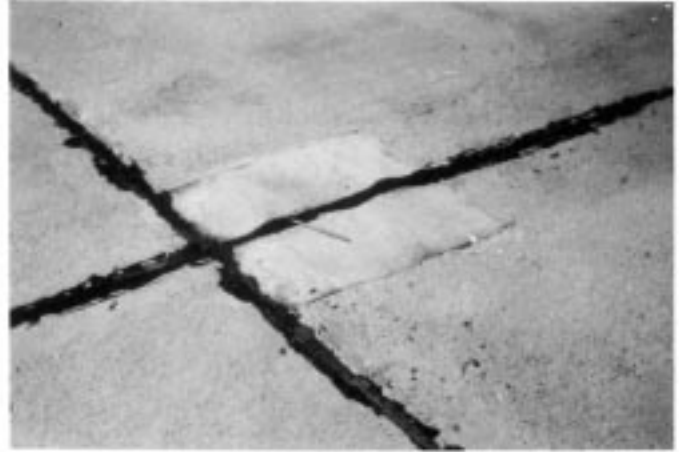
FIG. X2.28 Low-Severity Small Patch
