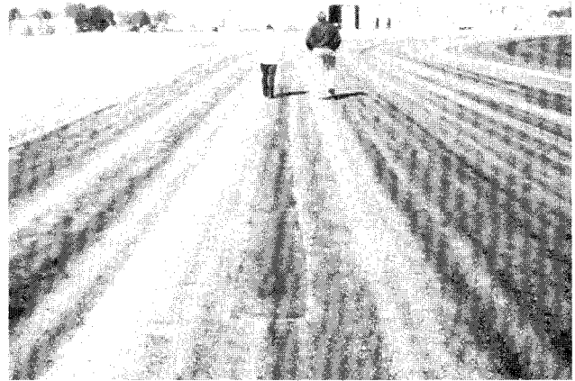
FIG. X1.48 Low-Severity Patch
