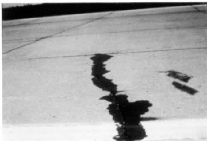
FIG. X2.13 Medium-Severity Transverse Crack
