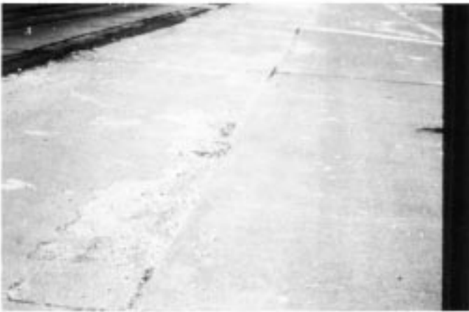
FIG. X2.46 High-Severity Scaling
