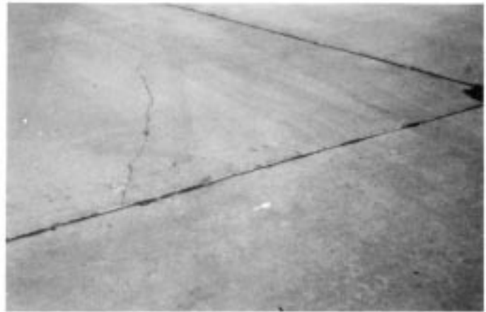
FIG. X2.11 Low-Severity Diagonal Crack
