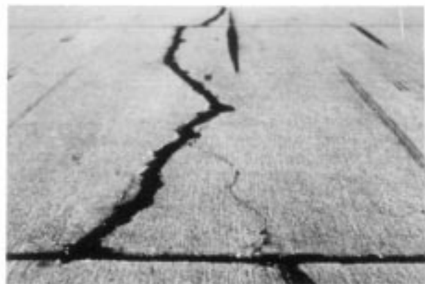
FIG. X2.16 High-Severity Longitudinal Cracks
