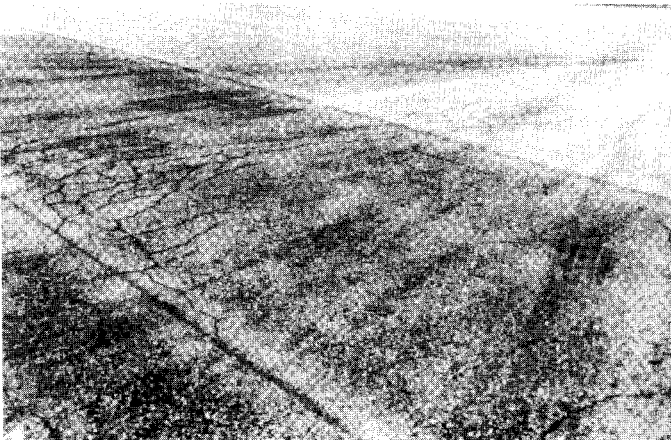
FIG. X1.8 Medium-Severity Alligator Cracking, Approaching High Severity (Example 2)
