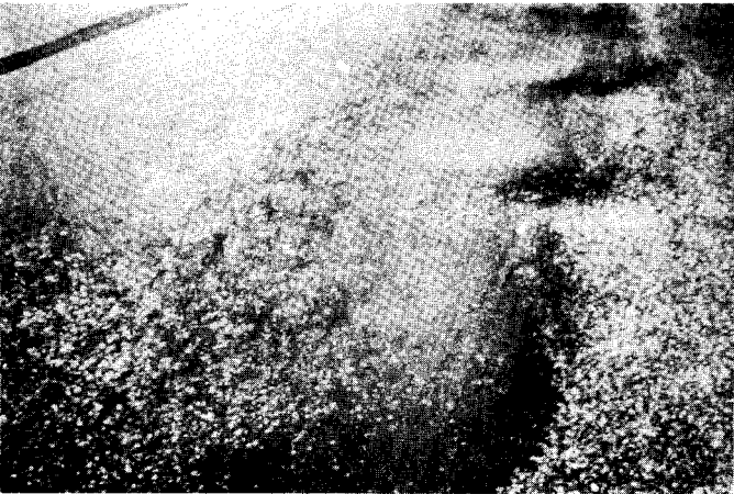
FIG. X1.23 High-Severity Corrugation
