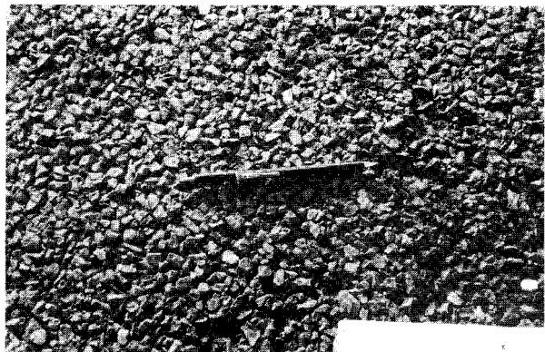
FIG. X1.63 Medium-Severity Raveling/Weathering on a Porous Friction Course Surface
