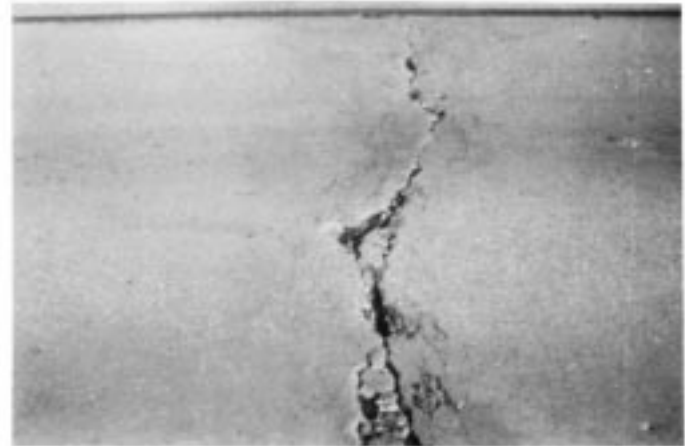
FIG. X2.15 High-Severity Crack
