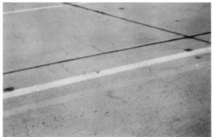
FIG. X2.60 Shrinkage Cracks
