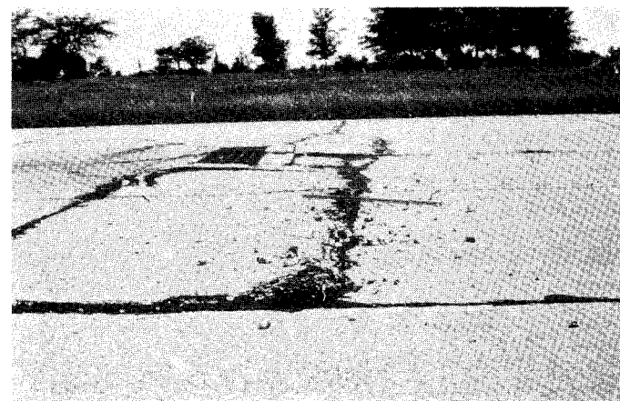
NOTE 1—This would only be considered low severity if the shattering in the foreground was the only part existing and the foreign material removed.
