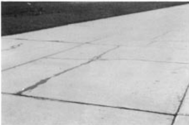
FIG. X2.57 Medium-Severity Intersecting Cracks
