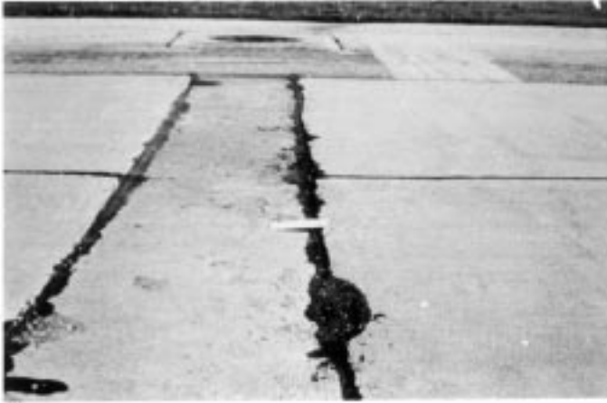
FIG. X2.36 Medium-Severity Utility Cut
