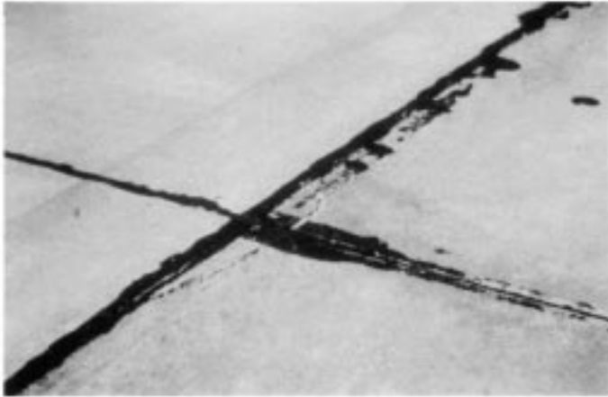
FIG. X2.70 Low-Severity Corner Spall
