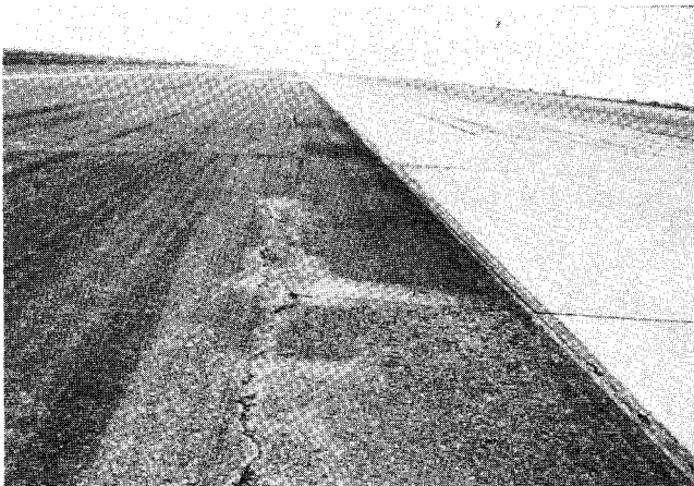
FIG. X1.41 Medium-Severity Longitudinal Crack
