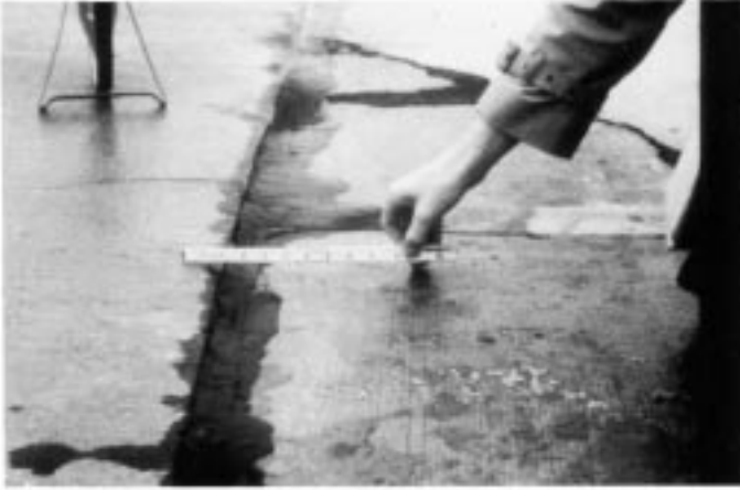
FIG. X2.51 Medium-Severity Settlement on Apron (>½ in. (13 mm))
