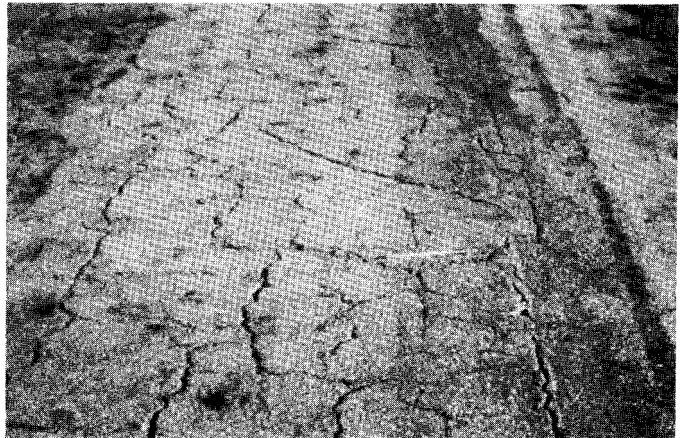
FIG. X1.20 High-Severity Block Cracking
