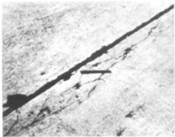
FIG. X2.20 Medium-Severity "D" Cracking
