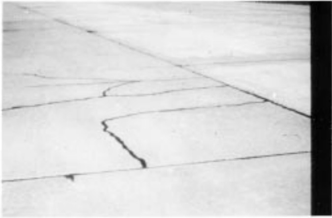
FIG. X2.55 Low-Severity Intersecting Cracks
