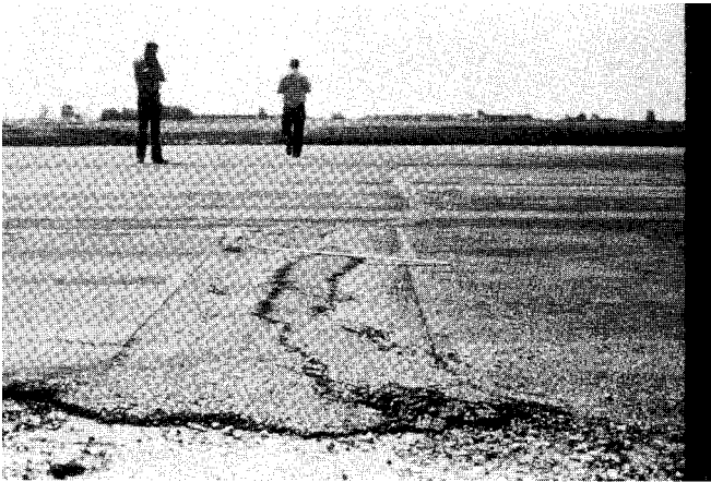
FIG. X1.52 High-Severity Patch
