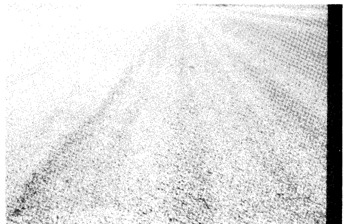
FIG. X1.54 Low-Severity Raveling/Weathering
