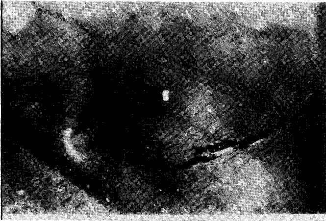
FIG. X1.74 Slippage Cracking
