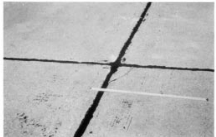
FIG. X2.69 Low-Severity Corner Spall
