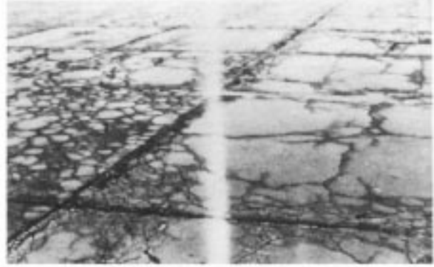
FIG. X2.48 High-Severity Scaling Caused by Alkali Aggregate Reaction
