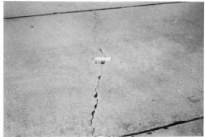
FIG. X2.14 Medium-Severity Transverse Crack
