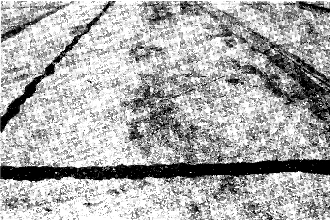
FIG. X1.31 Low-Severity Joint Reflection Cracking, Filled Crack
