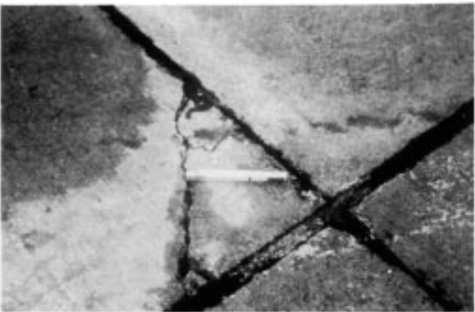
FIG. X2.71 Medium-Severity Corner Spall
