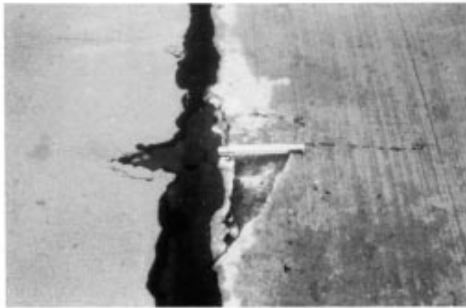
FIG. X2.66 Medium-Severity Joint Spall
