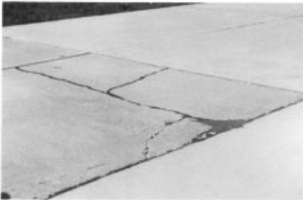
FIG. X2.56 Medium-Severity Intersecting Cracks
