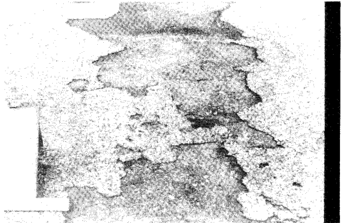
FIG. X1.59 High-Severity Raveling/Weathering
