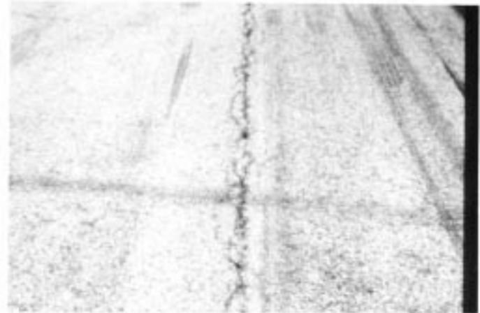
FIG. X1.39 Medium-Severity Longitudinal Construction Joint Crack
