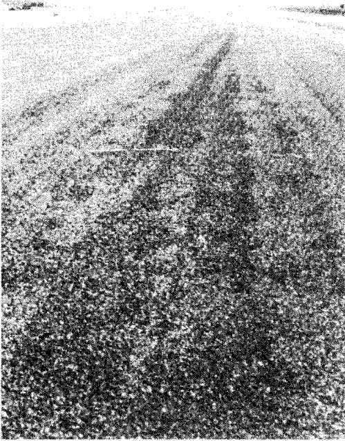
FIG. X1.64 Medium-Severity Raveling/Weathering Showing Rough and Pitted Surface
