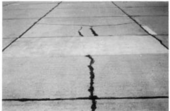
FIG. X2.34 Low-Severity Patch
