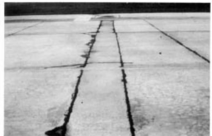
FIG. X2.35 Low-Severity Utility Cut
