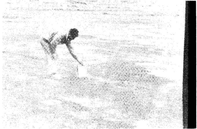
FIG. X1.58 High-Severity Raveling/Weathering
