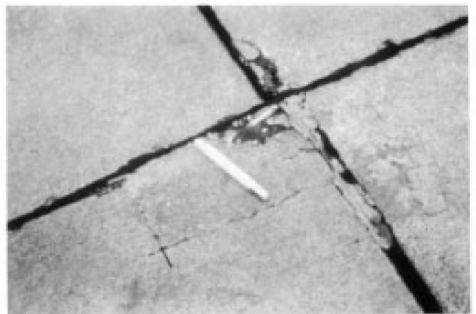
FIG. X2.30 Medium-Severity Small Patch
