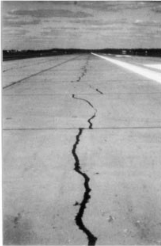
FIG. X2.12 Medium-Severity Longitudinal Crack
