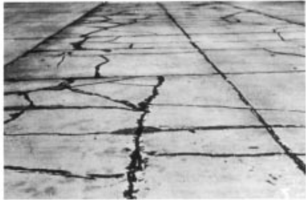
FIG. X2.58 Shattered Slab
