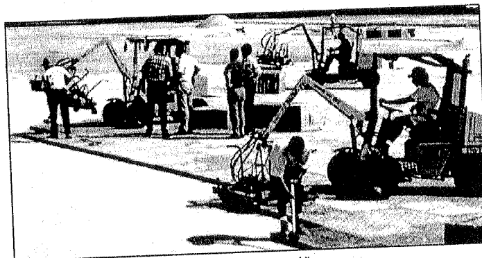
Mechanical installation equipment places concrete pavers rapidly.
