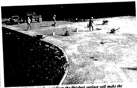
Figure 12. Excess sand swept from the finished surface will make the pavement ready for traffic.
