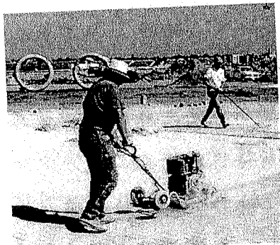
Figure 11. Vibrating sand into the joints.
