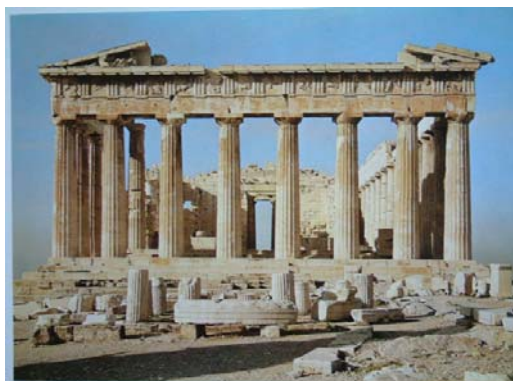
圖 28. Entasis: thickest at the point one-third from the base, then taper to the top
