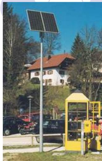
A telephone booth supplied by photovoltaics with an energy management system
