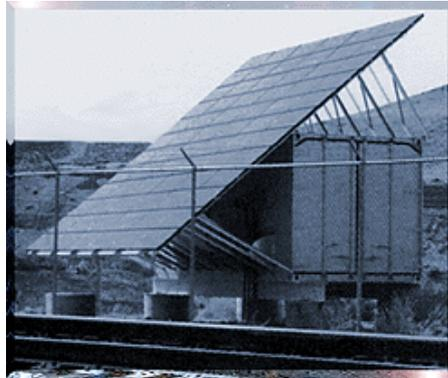
At Sand Pass in Nevada, 72 PV modules (60 W each), two propane-powered generators, and a large battery bank operate together to improve the economics and reliability of a remote telephone signal booster station. (Photo: Northern Power Systems)
