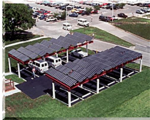
This electric vehicle recharging station in southern Florida is powered by a grid-connected PV array mounted on the roof. When no vehicles need charging, power from the modules is transferred to the utility line. (Photo: University of South Florida)
